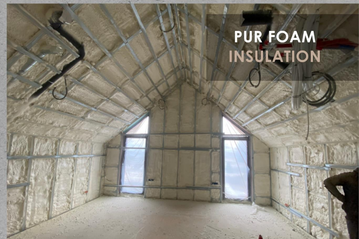
EXECUTION OF INDOOR INSTALLATIONS
