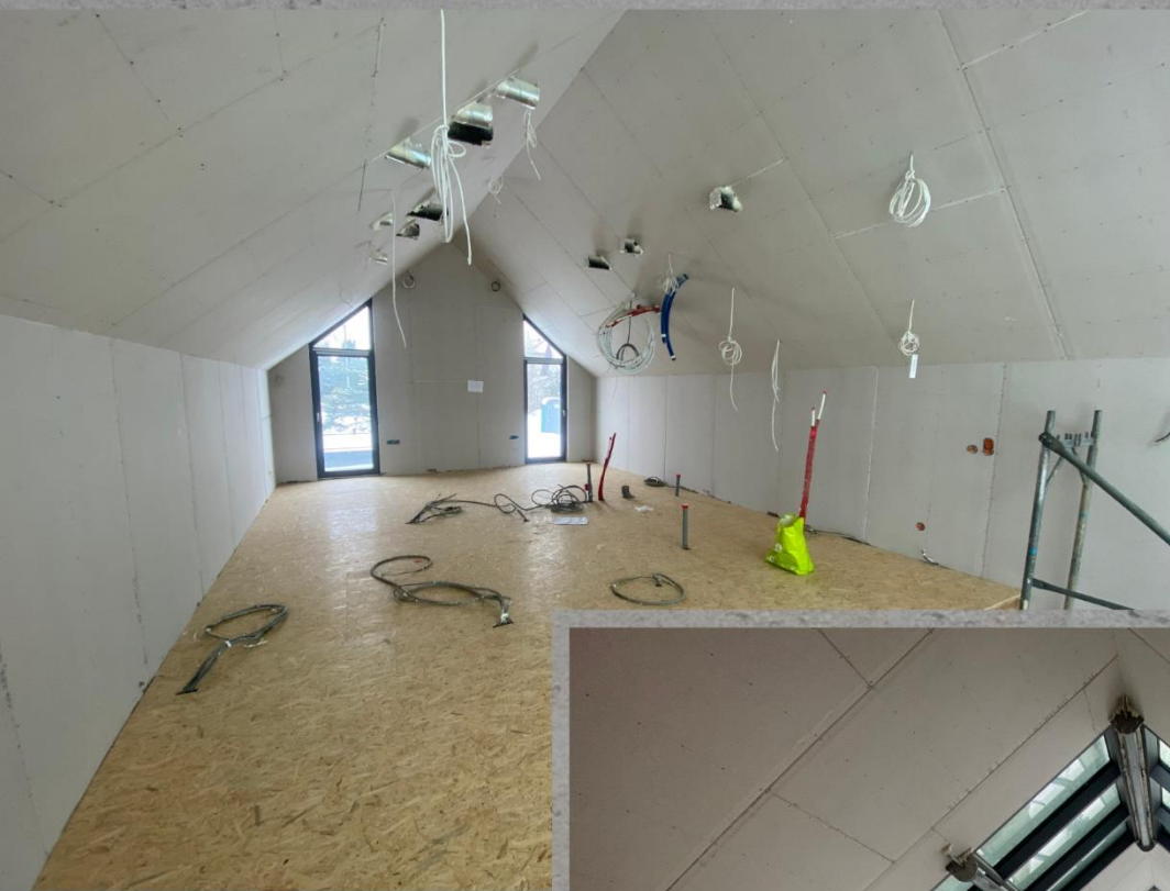
MONTAGE OF PLASTERBOARD AND PULLING OUT THE INSTALLATIONS
