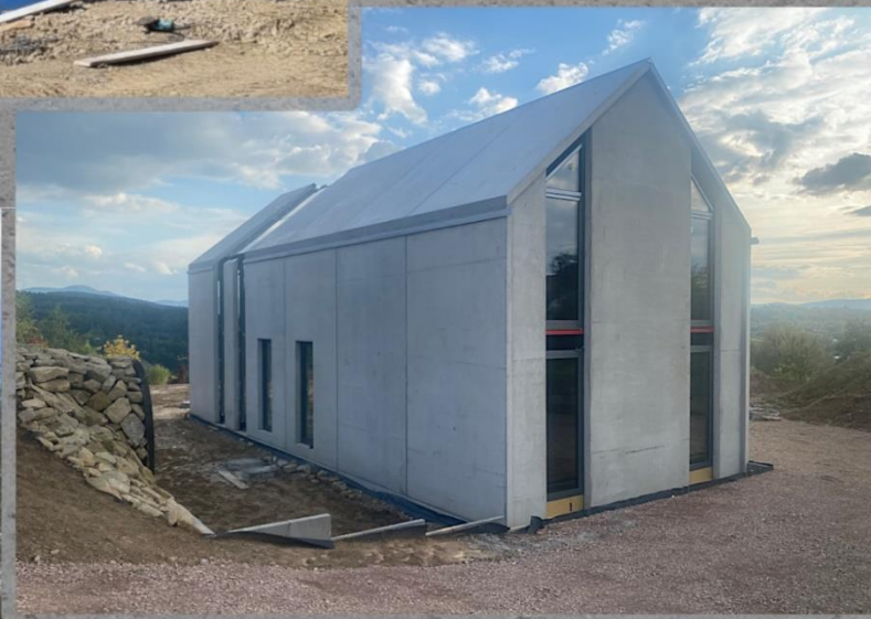
MONTAGE OF WINDOW JOINERY
