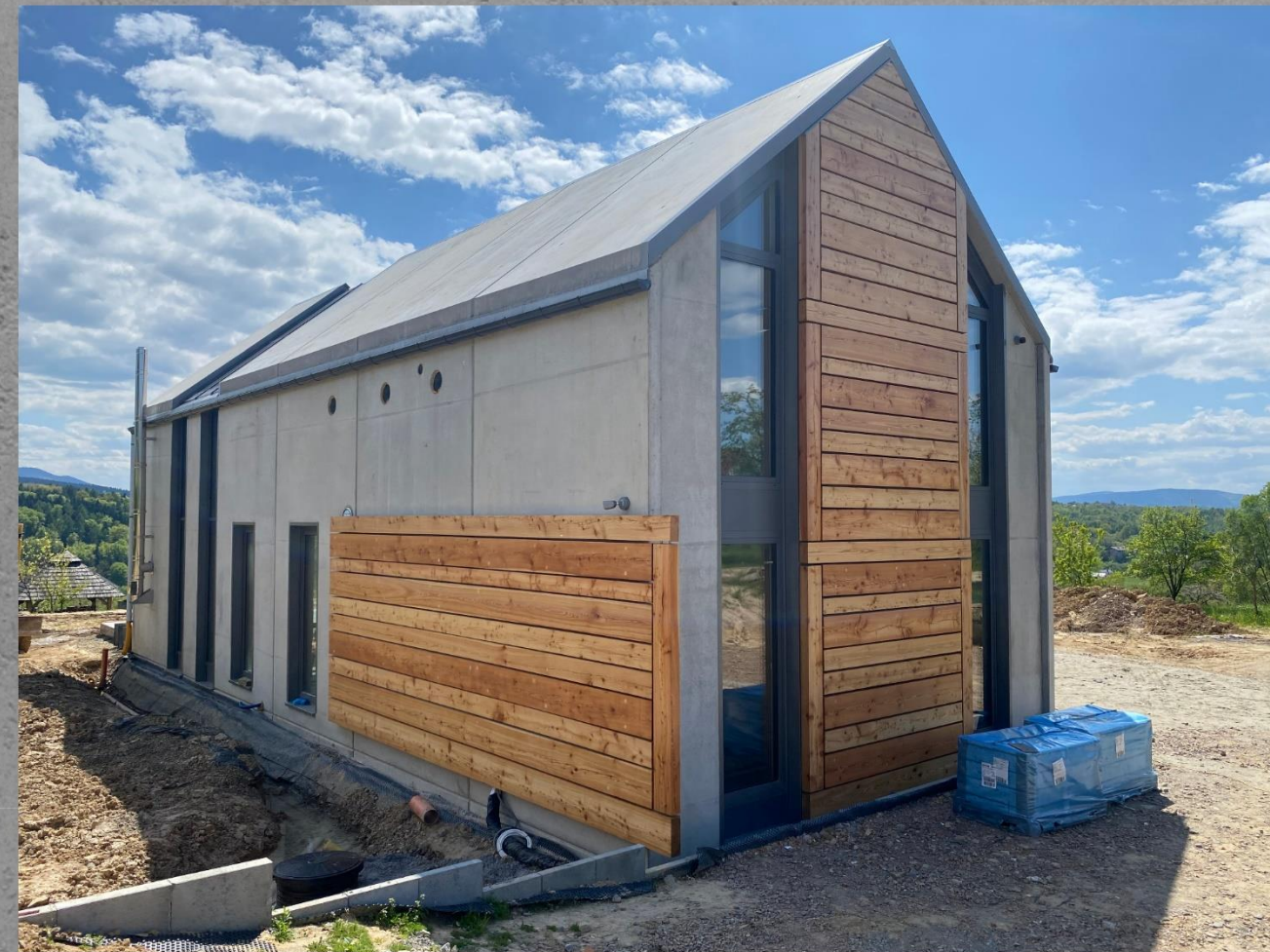
EXECUTION OF DECORATIVE FACADE ELEMENTS - TIMBER
